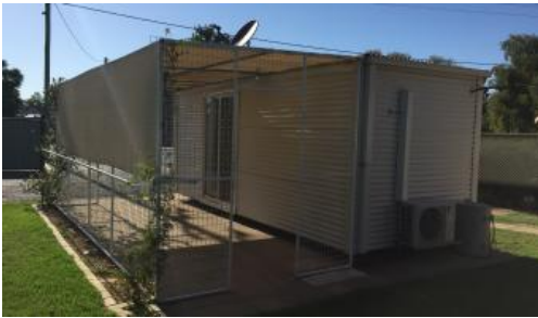
Site 2, 2-6 Warrabungle St, Gunnedah
