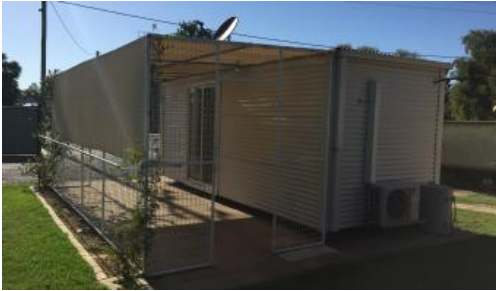
Site 2, 2-6 Warrabungle St, Gunnedah
